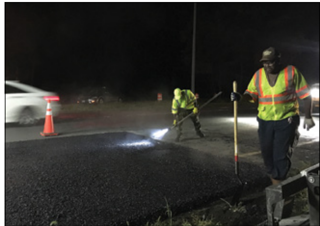
I-495 resurfacing in Montgomery County.
