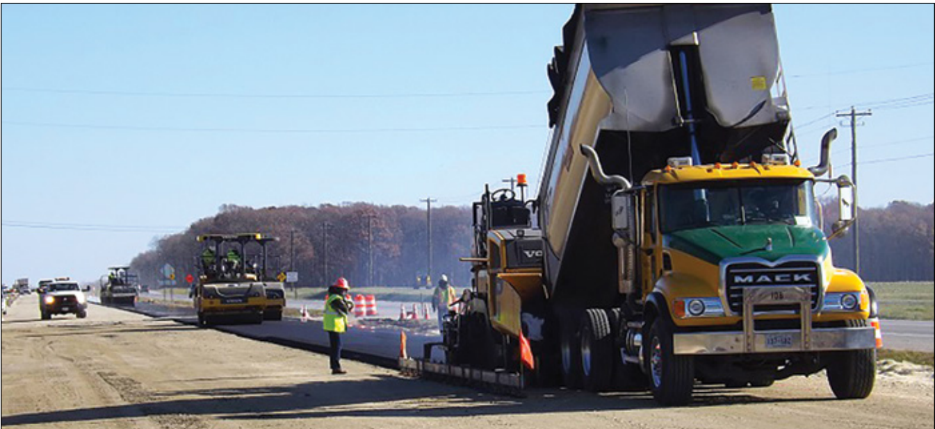
Progress on MD 404 near Church Lane.
