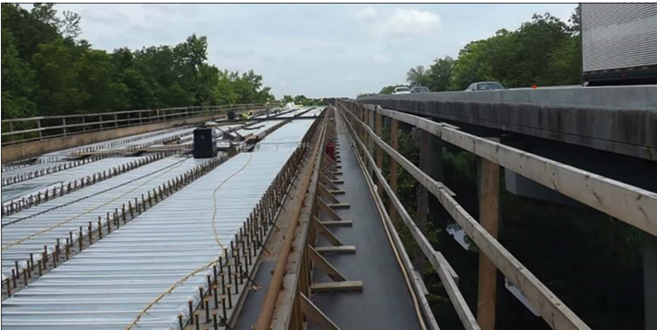
Southbound US 13 bridge.
