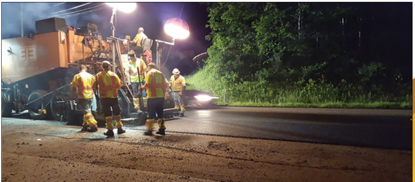
Crews applying ultrathin bonded wearing course on MD 36 in Allegany County.
