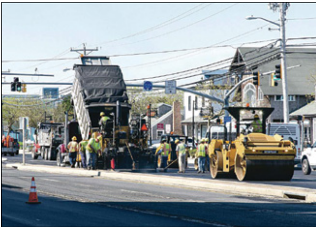
Coastal Highway (MD 528) resurfacing.
