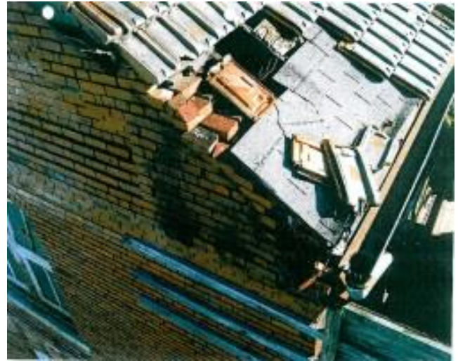
Above Left: Footer's Dye Works, southern perspective with sawtooth structures removed. Above Right: Roof tiles, several of which are missing. Below: FDW after "moth balling" was completed.
