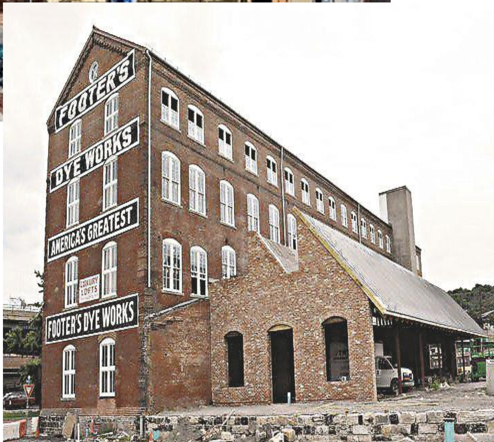
Right: FDW with new signage, windows and new sawtooth addition.
