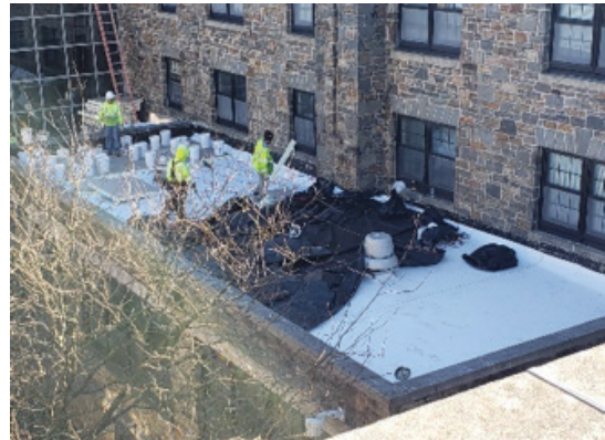
Harper Tubman House Roof
