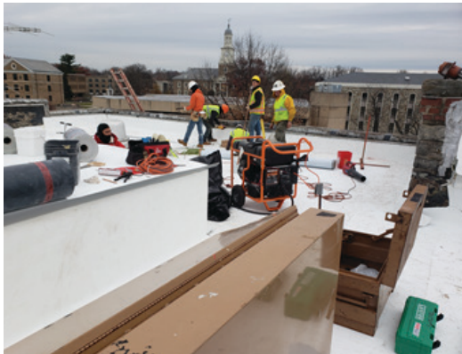
Baldwin Hall Roof
