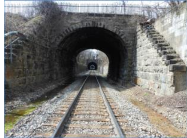
Guilford Ave Bridge Replacement
