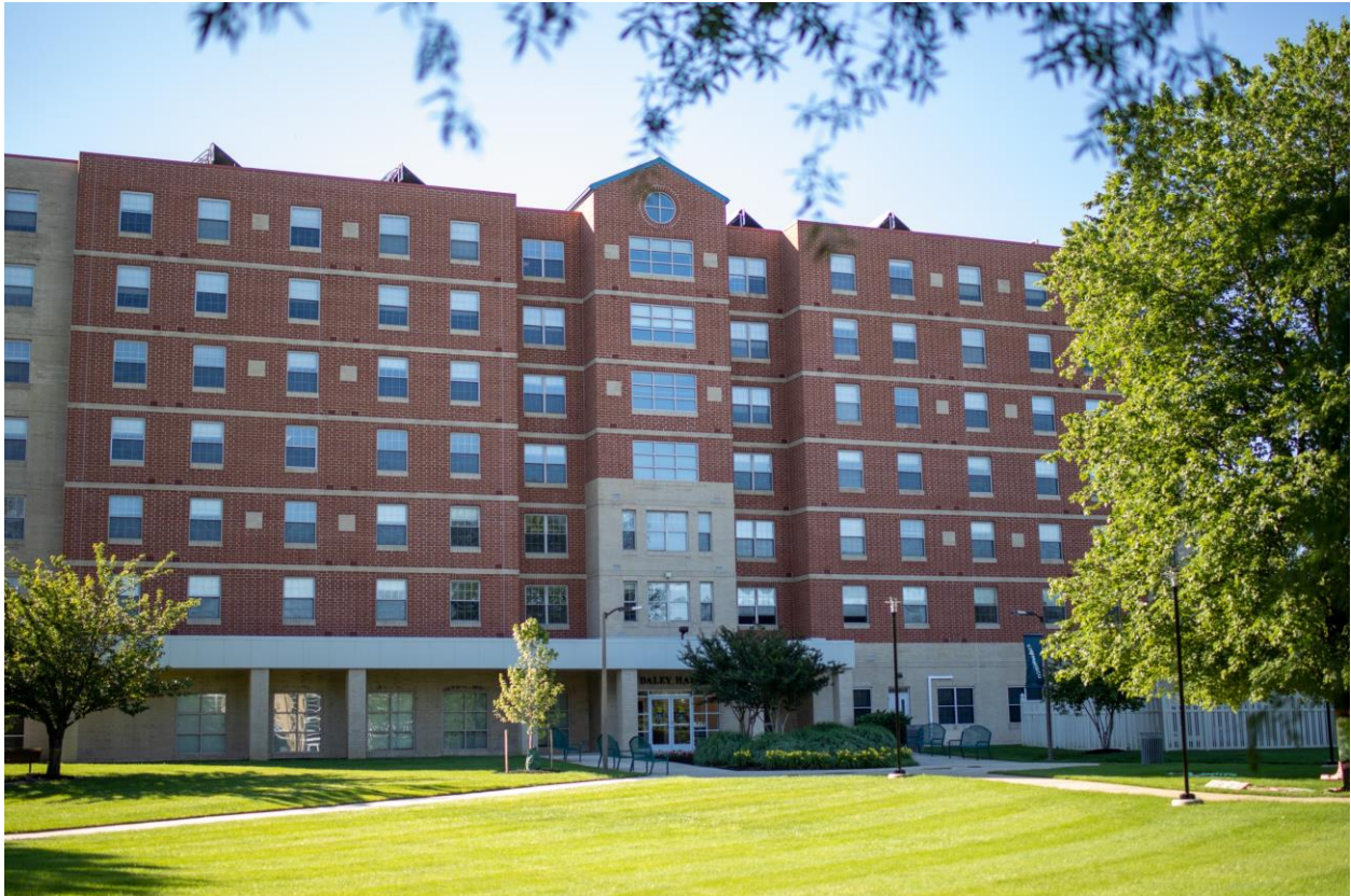
Daley Hall is one of two residency halls currently on Coppin's campus.
