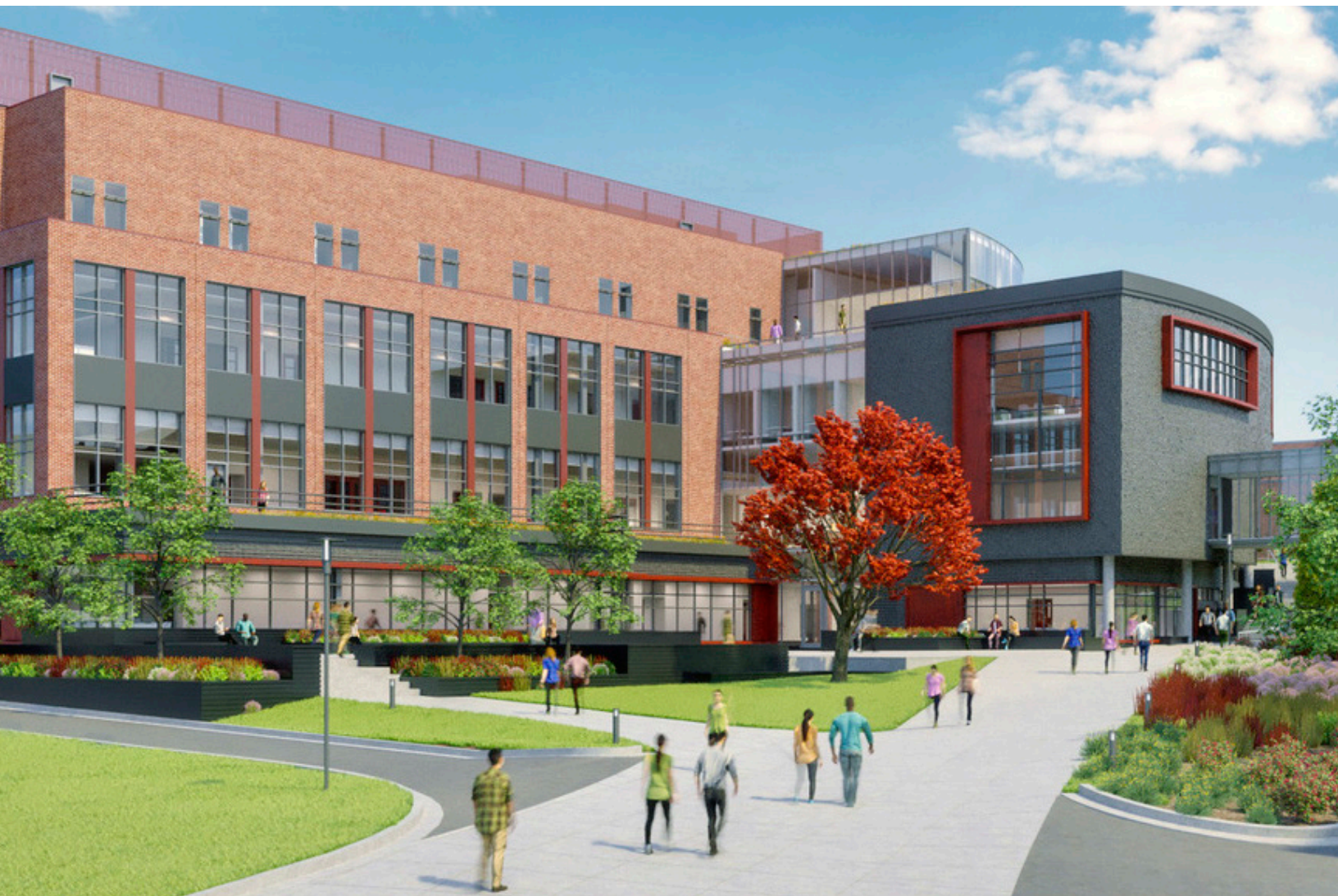
Design for Education & Health Sciences Center, shown under construction on cover.
