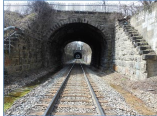
Guilford Ave Bridge Replacement
