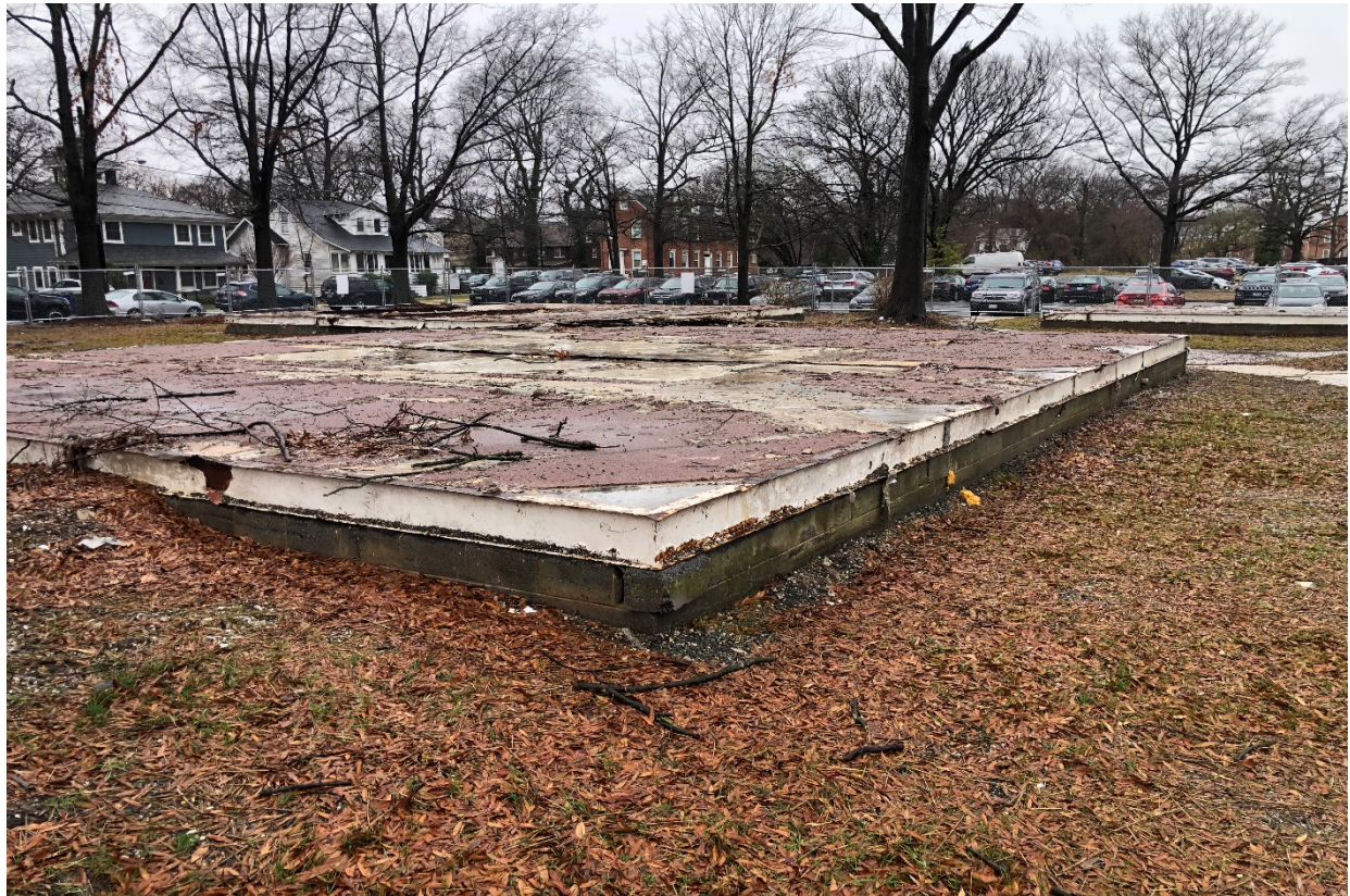
Demolished old housing on the proposed site
