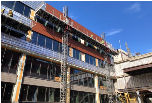
Above and right: Construction Progress
