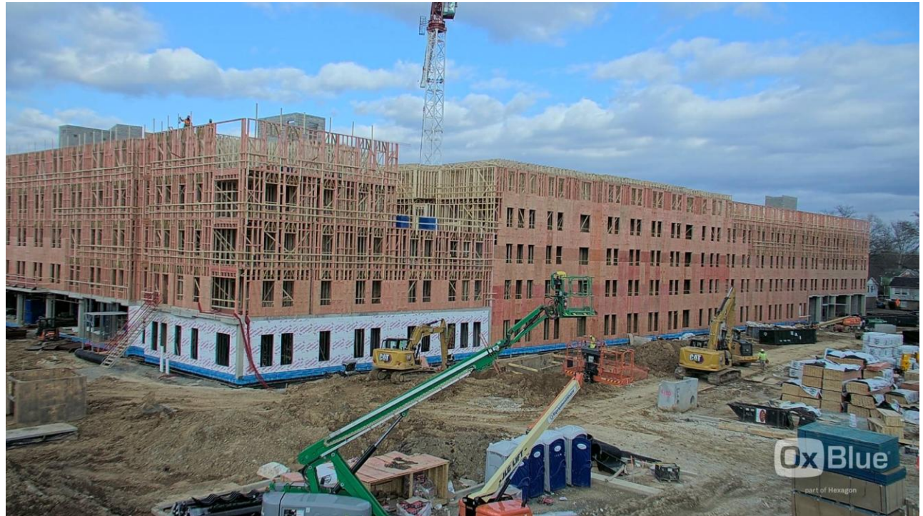
Current construction activity
