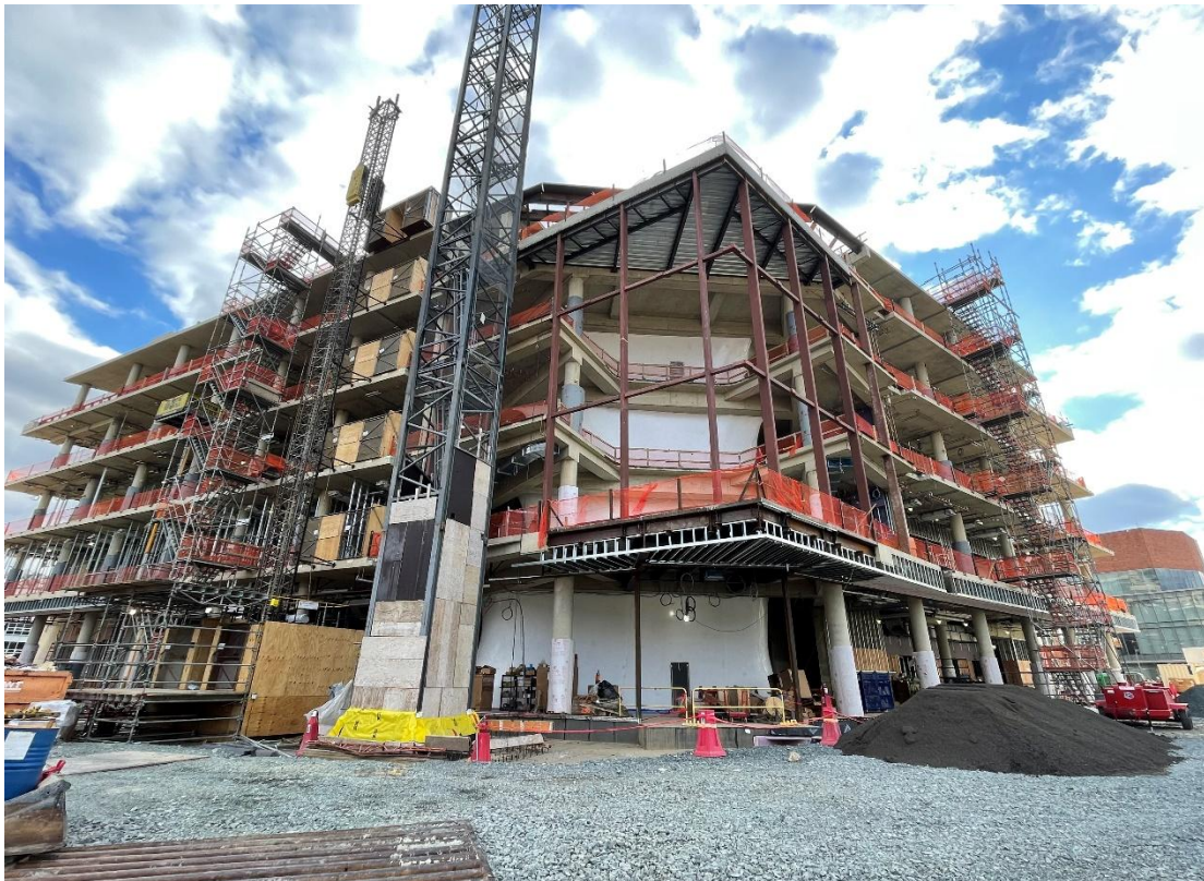
Current construction activity
