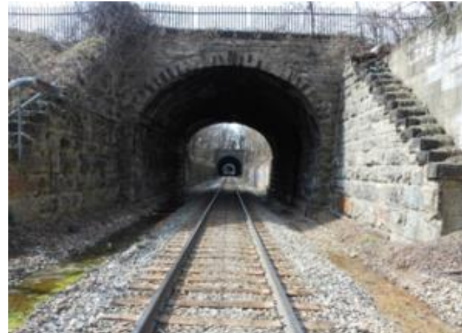
Guilford Ave Bridge Replacement
