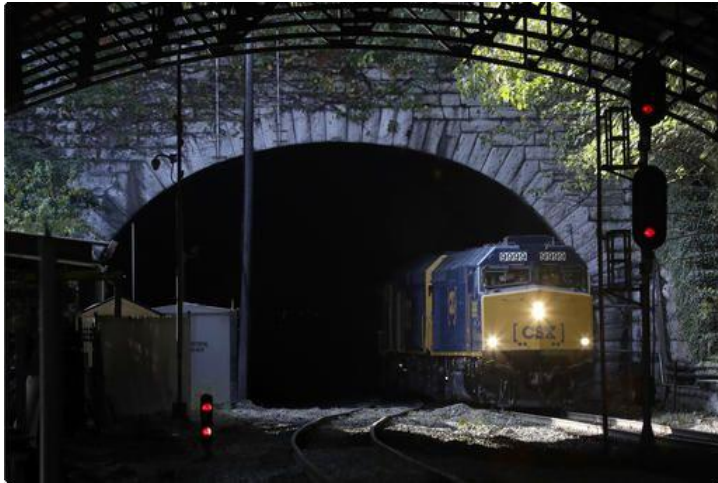
Howard Street Tunnel North Portal
